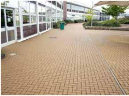
More concrete block permeable paving has recently been added to the original areas, serving additional buildings.
