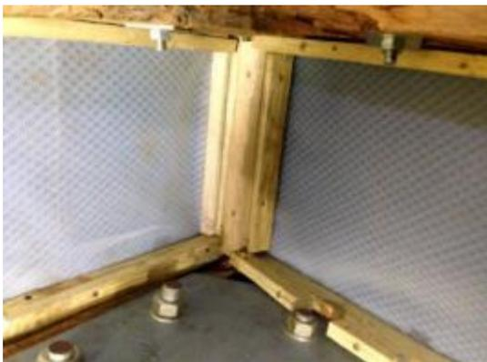
Fig 5. Overlain Netlon® with battens onto the BRM at Site 3.
