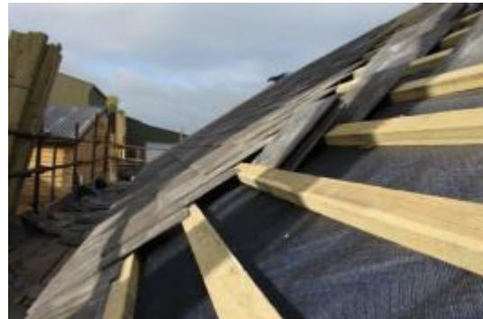
Fig 4. Overlaying battens and tiles over the Netlon® as part of the re-roofing works at Site 2.
