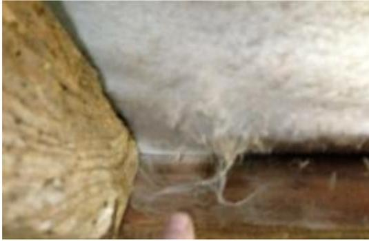
Fig 1 Fluffing and staining of BRM at Site 1.
