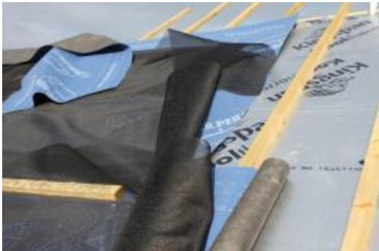
Fig 3. Overlaying the Netlon® onto the BRM at Site 2 as part of the re-roofing works.
